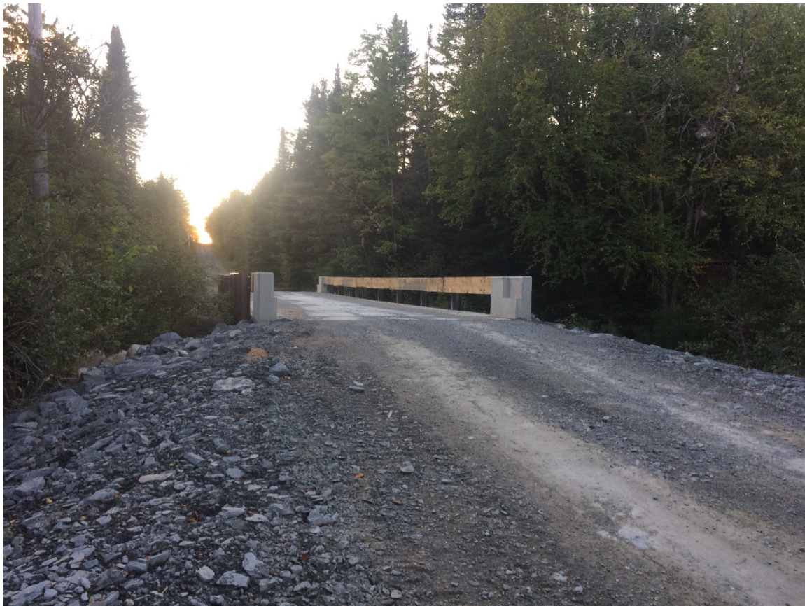
The newly replaced Slipp Road Bridge which was completed in 2017.
